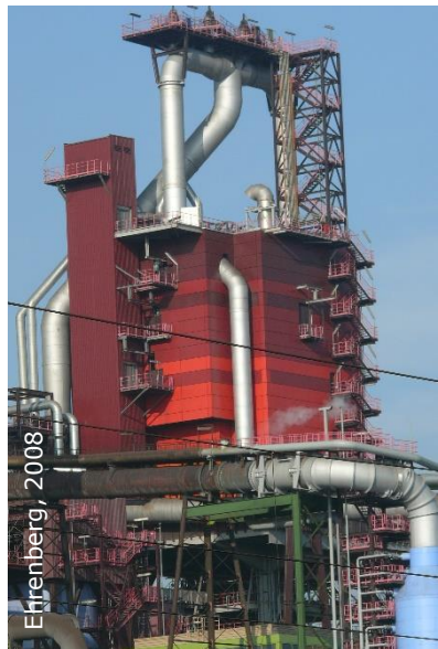
Blast furnace \approx 280 \text{ kg slag per ton}_{\text{HM}}
